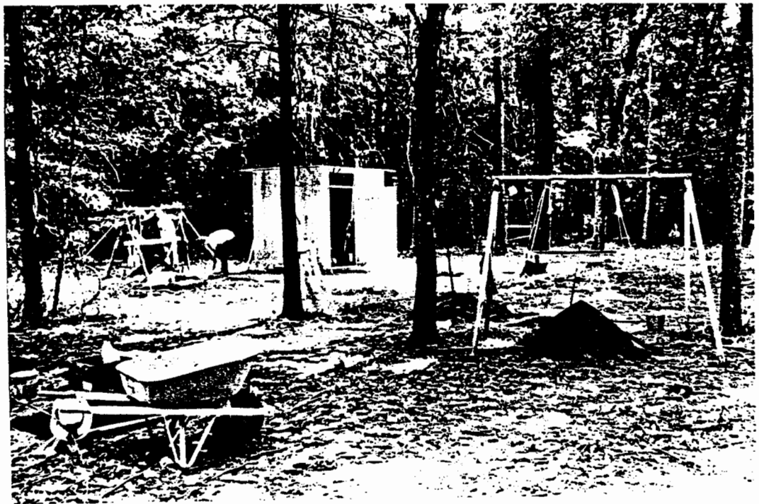
Figure 2-7. Random square excavations proceeding in the vicinity of the equipment storage shed, at the northern end of the site. (Negative ).
