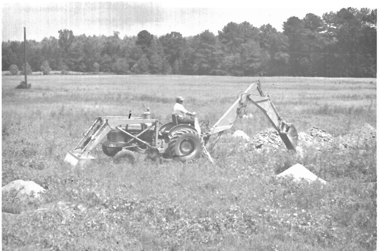
FIGURE 31 – Backhoe operations at Site 38LX82. A 30 meter trench was opened through the center of maximum artifact concentration in an unsuccessful attempt to locate subplowzone features.
